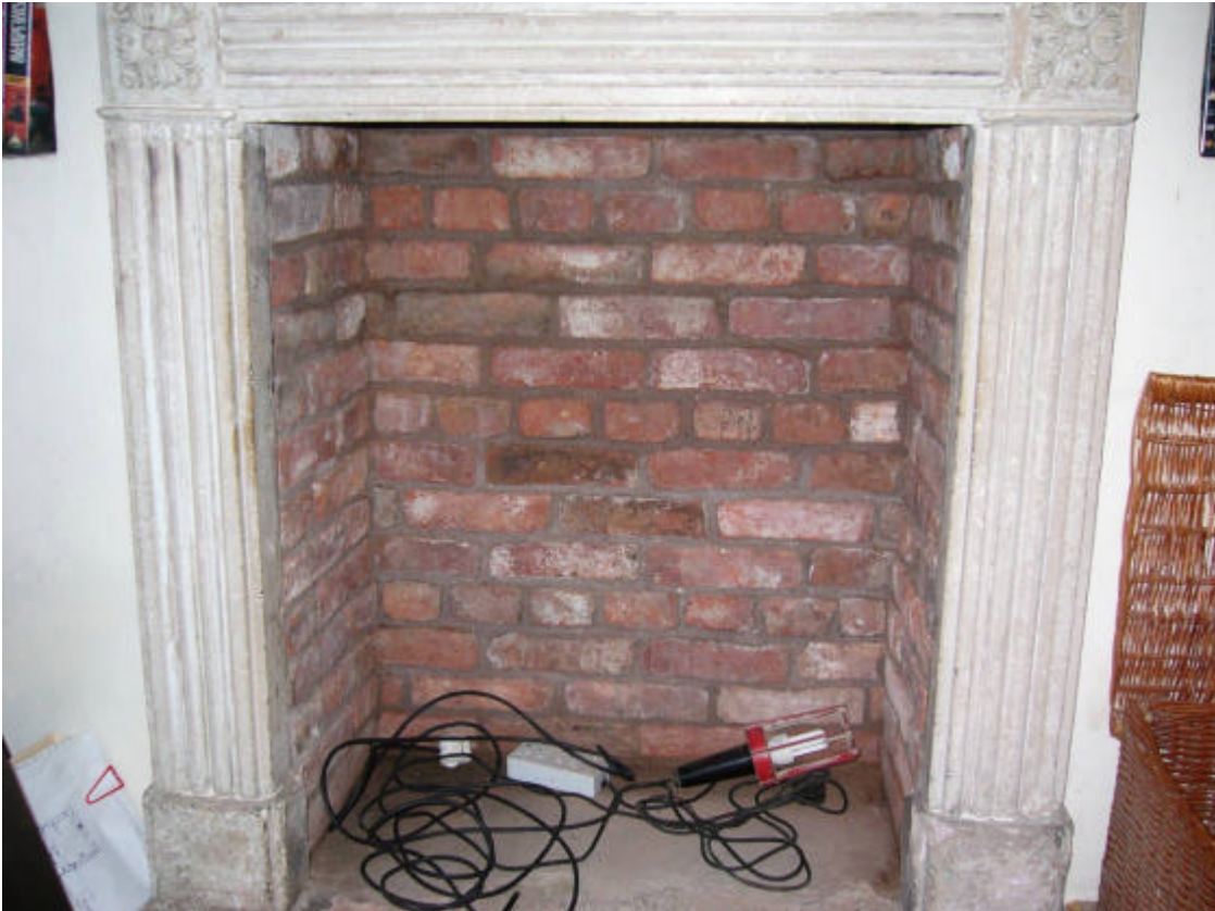
Figure 2. The new hearth and stripped fire surround.
