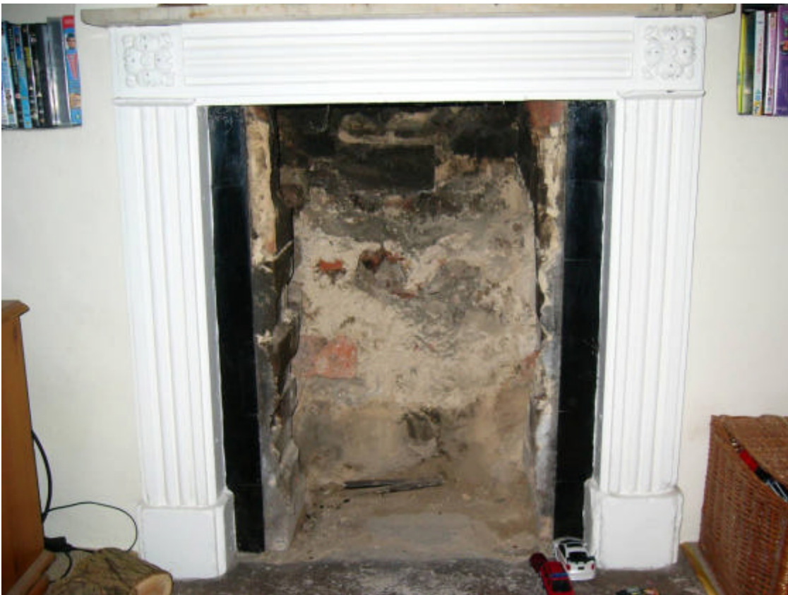
Figure 1. The original fireplace and rubble fill.
