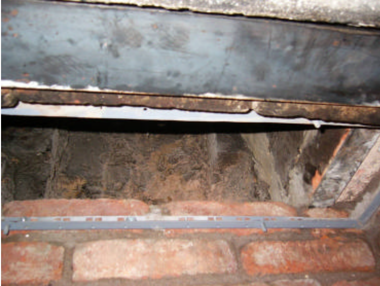
Figure 3. The register plate frame.
